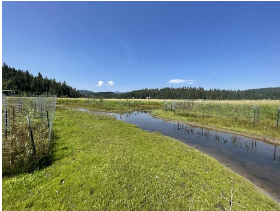
New channel of Cougar Creek looking south.
